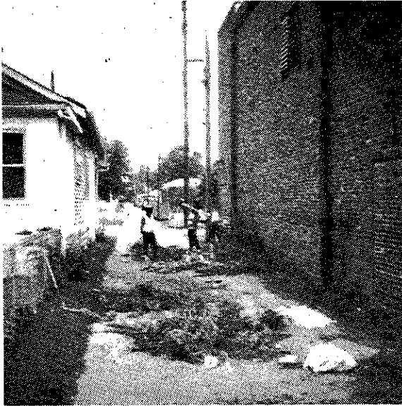
The Youth Workers cleaning an alley.
