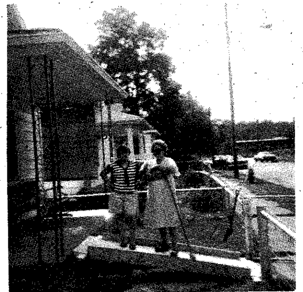
The much needed ramp.
